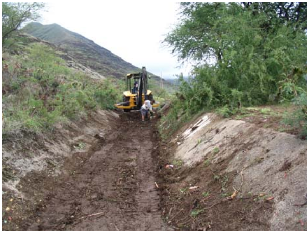
Juan Garcia in drainage area
