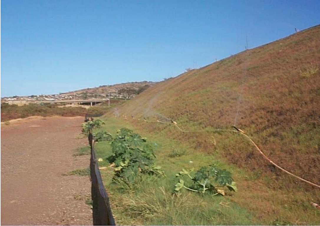
Slope protection BMP
