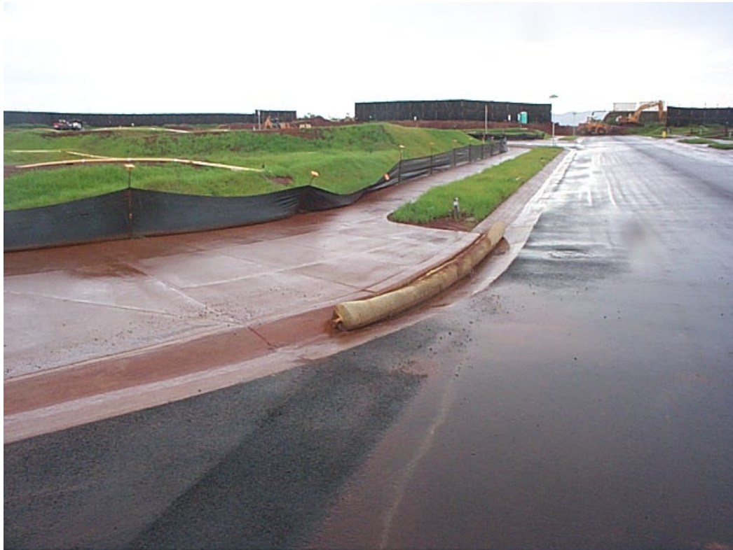
Inlet protection and silt fence
