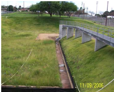
Drainage detention basin
