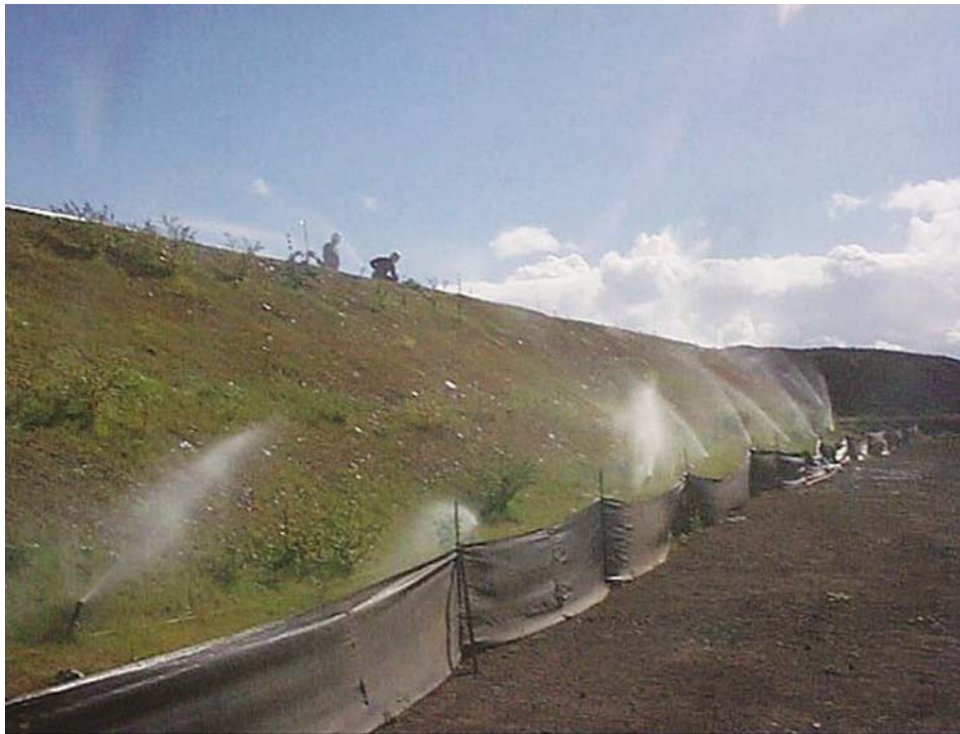
Slope stabilization and silt fence
