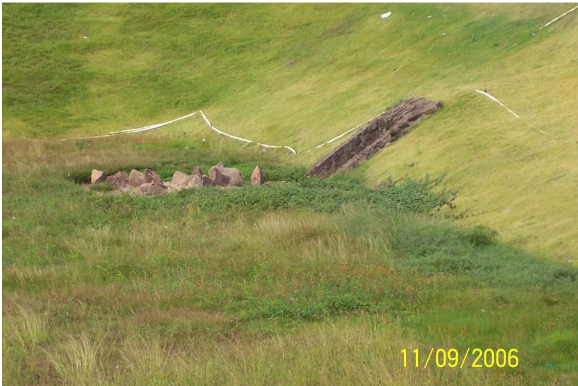
Drainage detention basin
